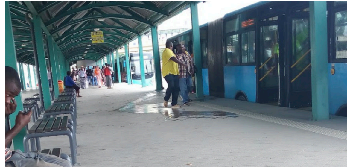
Img. 69: Ubongo terminal from the inside
