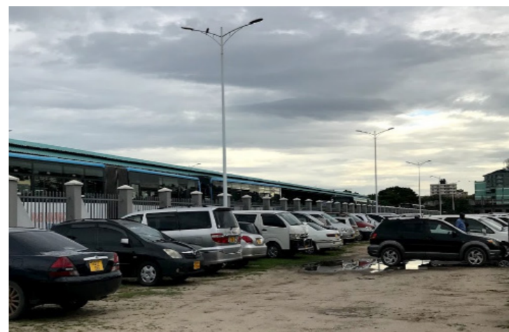
Img. 64: Unproper accesibility BRT Terminal
