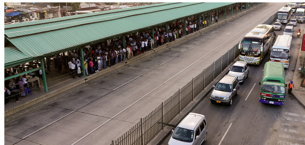
Img. 71: Kimara terminal
