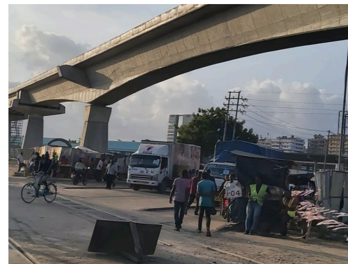
Img 56: Lack of transfer structures between BRT and railway
