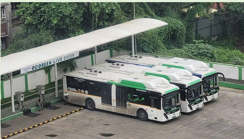
Charging Infrastructure at Pune Railway Station Depot
