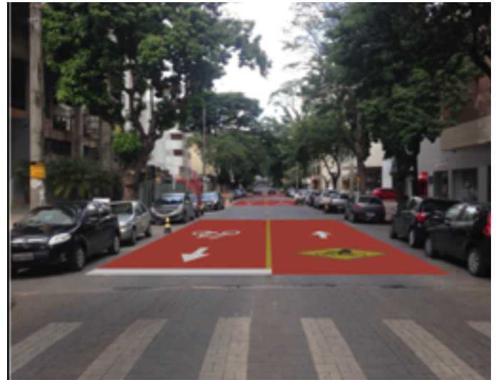
Figure 3: Horizontal signaling for the Fahrradstraße
